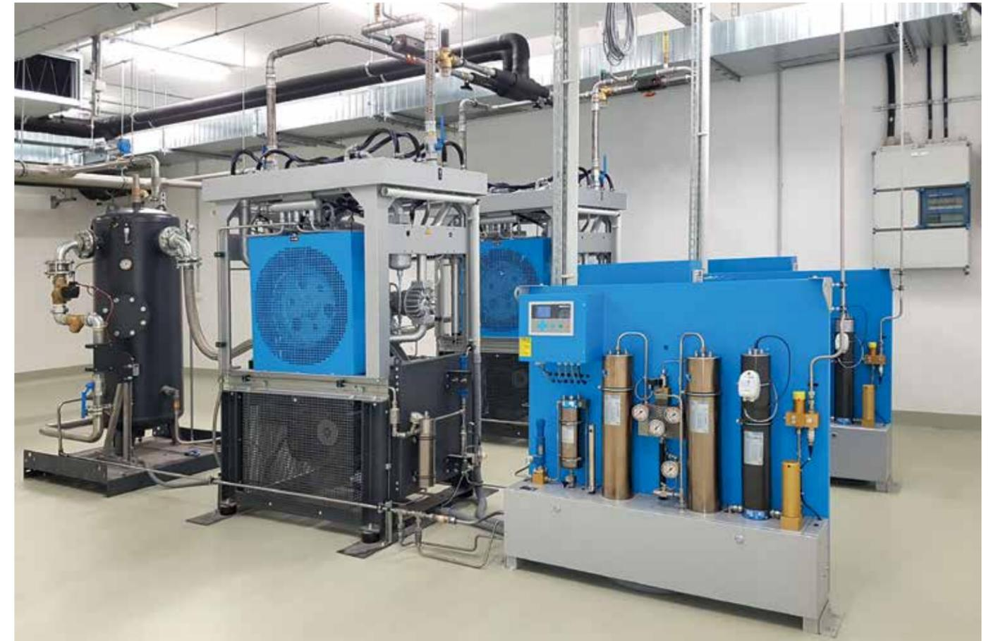
Vertical 40HP GR23 series high-pressure helium compressor, available air-cooled or water-cooled with inlet buffer tank and gas purifier/dryer.
