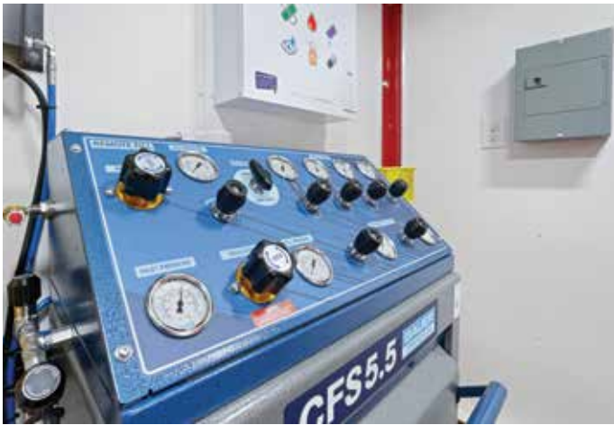
› The SCBA rack has space for 14 spare bottles. Built-in cabinets can hold spare SCBAs, masks, parts, first-aid kits, Haz Mat gear, communication equipment, and more. Electrical power assures that all battery-operated devices can be fully charged.
